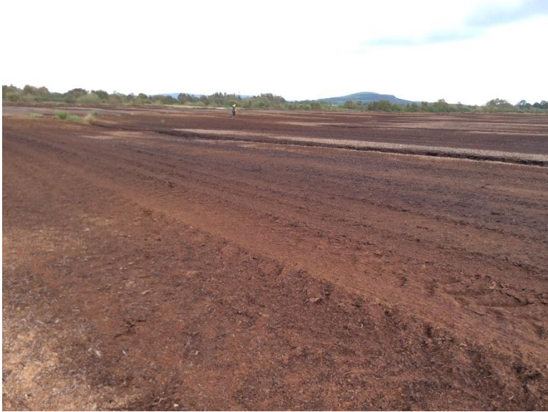
Plate 40: General view of hardstand for T10 (2020), looking NE.
