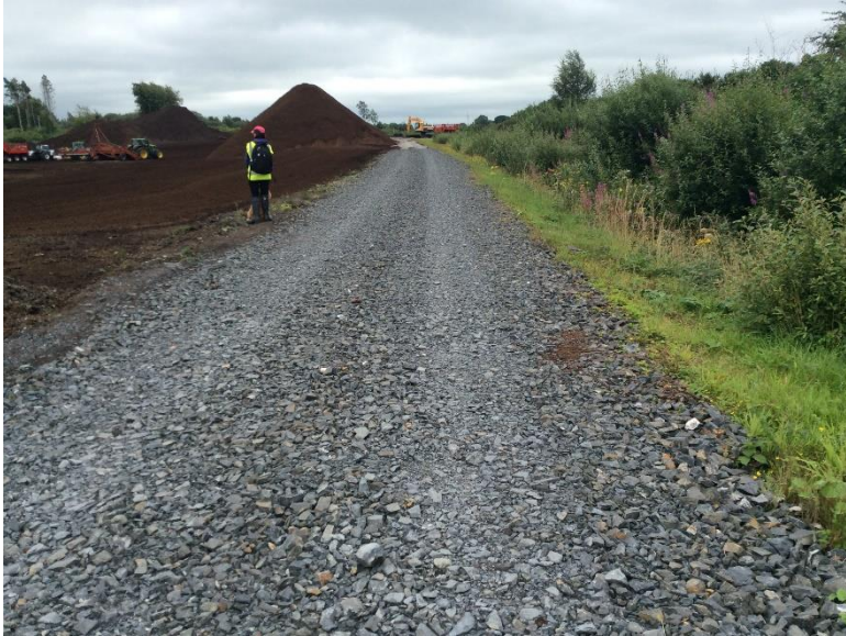
Plate 34: Existing track due for upgrade between T8 and T9 (2016), looking SE.
