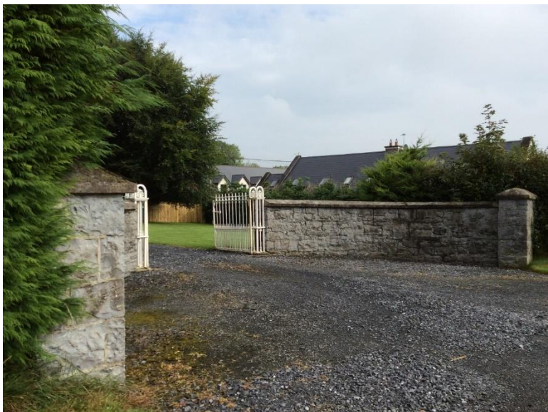
Plate 83: Stone wall, piers and cast iron gates at entrance to NIAH 15401915 at Irishtown townland along proposed Grid Connection Route.
