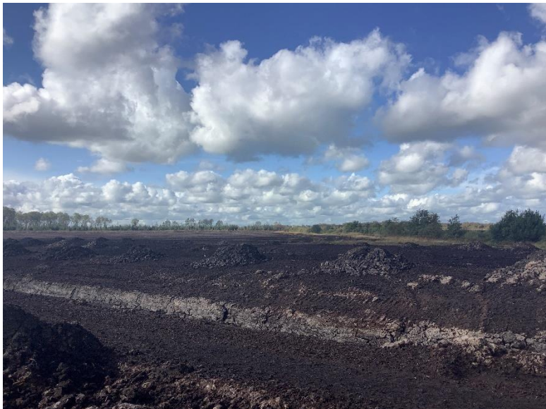
Plate 5: General view of T2 and associated hardstand (2020), looking WSW.
