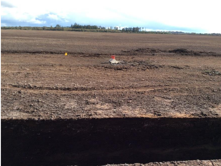
Plate 28: Proposed location of turbine base for T7, looking SE.
