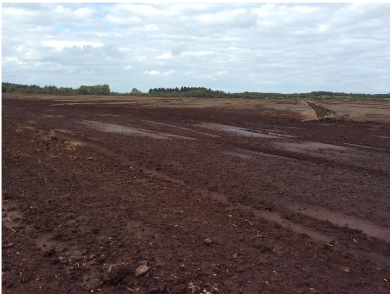
Plate 41: General view of proposed location of T11 and associated hardstand, looking NW.
