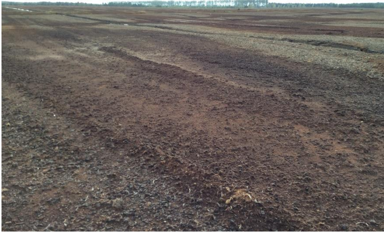
Plate 38: General view of access track to T10 (2020), looking SW.
