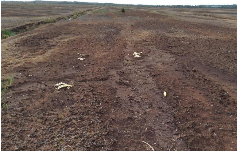
Plate 48: General view of NE end of proposed access track to T12, looking SW.
