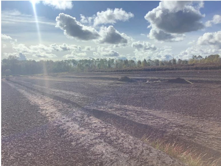
Plate 2: T1 (2020), looking SW towards turbine base and hardstand.
