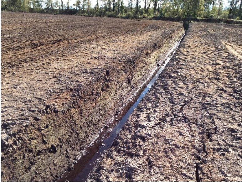
Plate 10: Drain faces in area of hardstand, looking SW.
