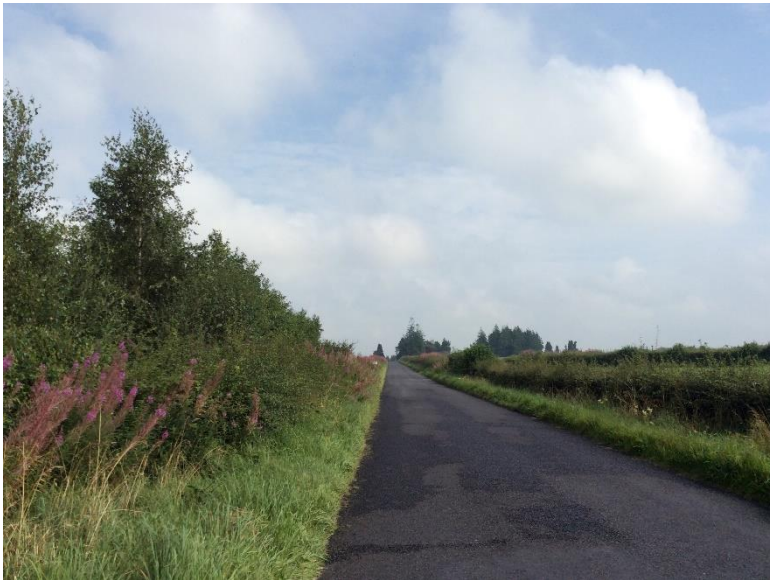
Plate 91: General view of proposed Grid Connection Route along public road at Clonva td.
