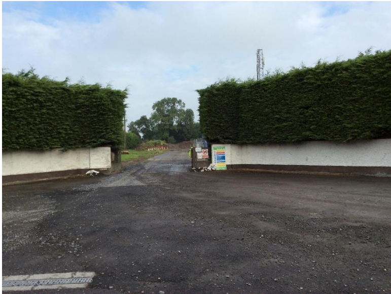
Plate 82: Entrance to existing Mullingar substation.
