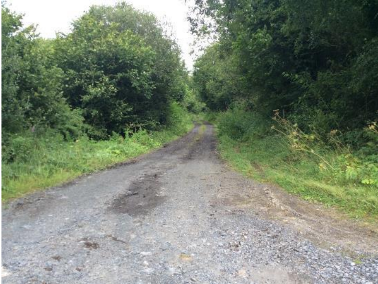
Plate 20: Existing access track to SW of T5, looking NE.
