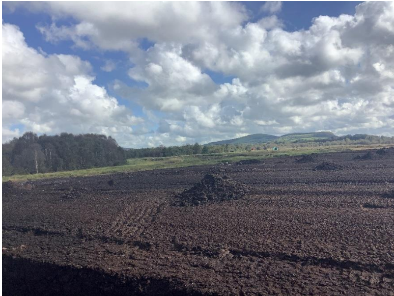
Plate 4: Eastern end of proposed hardstand area of T2 (2020), looking ESE.
