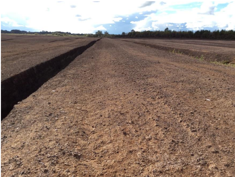
Plate 27: General view of T7 and associated hardstand, looking SW.
