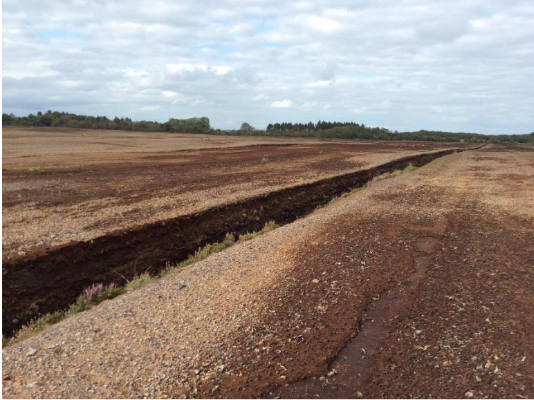
Plate 42: Hardstand and turbine base (2020), looking NNE.
