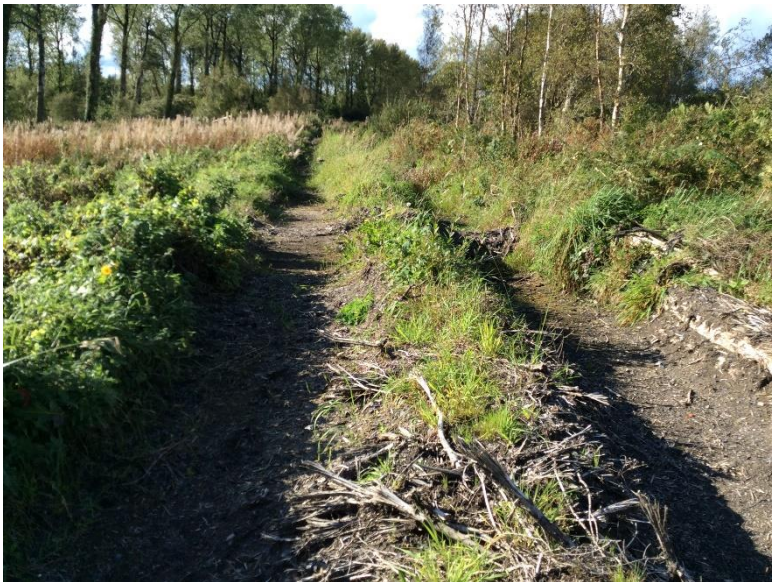
Plate 15: Existing track due for upgrade to SE of T3, looking NW.
