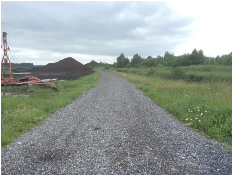
Plate 7: Existing road due for upgrade between T2 and T4, looking north-west.
