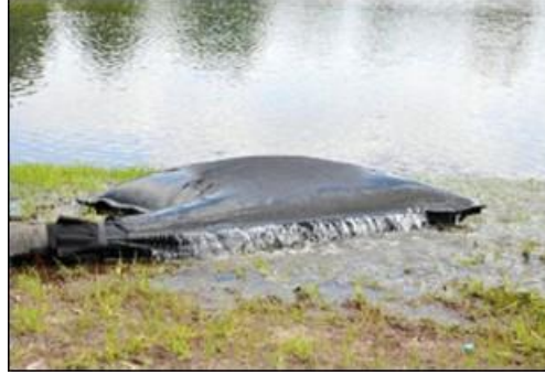
Plate 4-7 Silt bag under inspection
