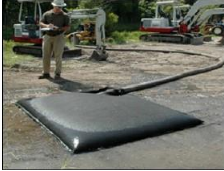
Plate 4-6 Silt Bag with water being pumped through
