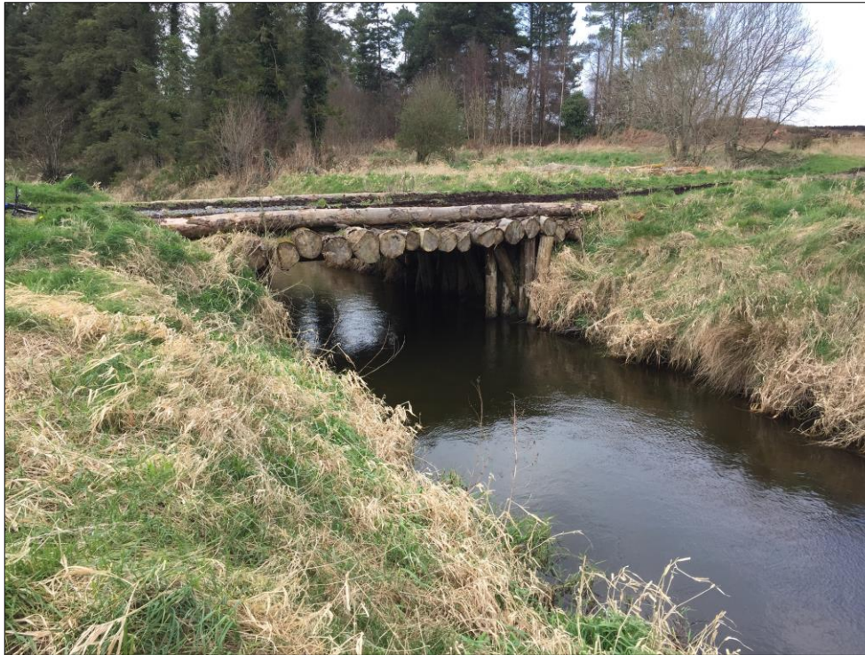
Plate 4-8 Existing timber bridge crossing on River Glore, proposed to be replaced
