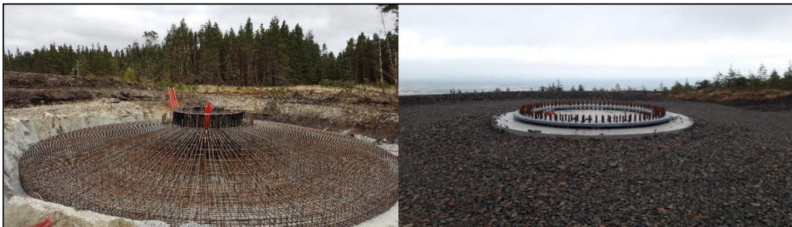
Plate 4-2 Turbine 'Anchor Cage' and finished turbine base
