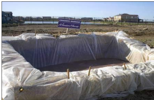
Plate 4-3 Concrete washout area
