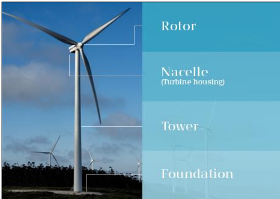
Plate 4-1 Wind turbine components
