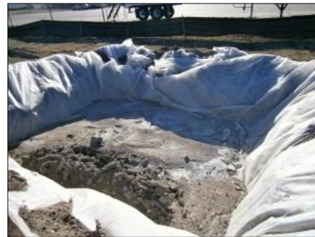
Plate 4-4 Concrete washout area
