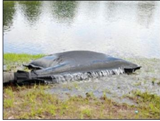
Plate 4-2 Silt bag under inspection
