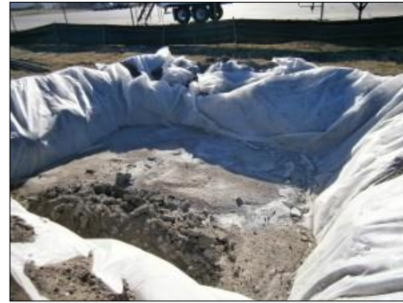
Plate 44 Concrete Wash Out Area
