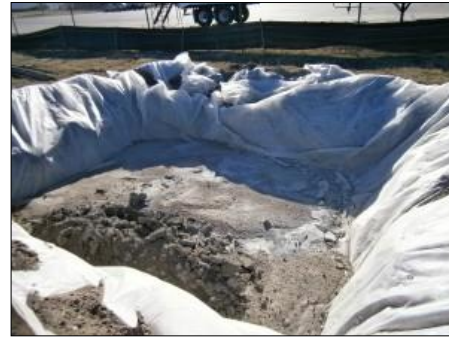
Plate 44 Concrete Wash Out Area
