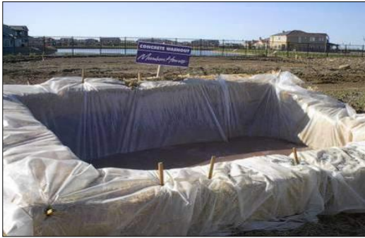
Plate 43 Concrete Wash Out Area
