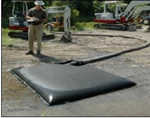
Plate 4-1 Silt Bag with water being pumped through
