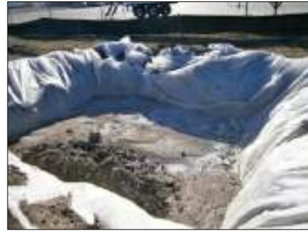
Plate 44 Concrete Wash Out Area
