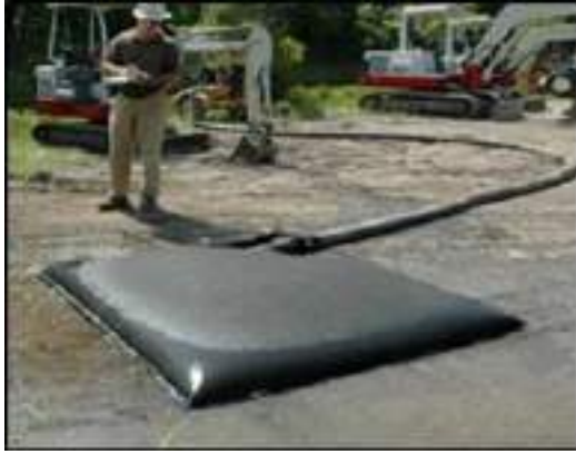
Plate 4-1 Silt Bag with water being pumped through
