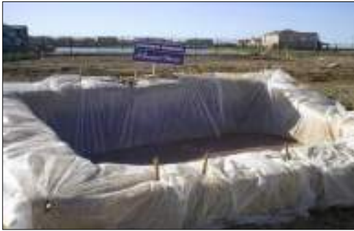
Plate 43 Concrete Wash Out Area
