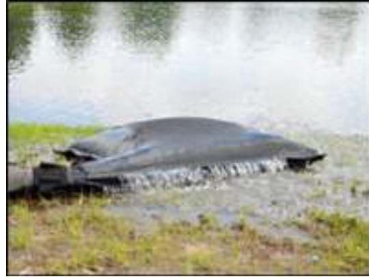
Plate 4-2 Silt bag under inspection
